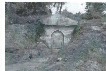
The Mausoleum slowly being revealed
